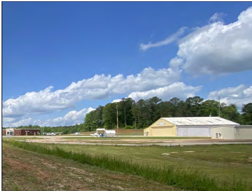
Figure 5.4. West view of airport office and hangars.
