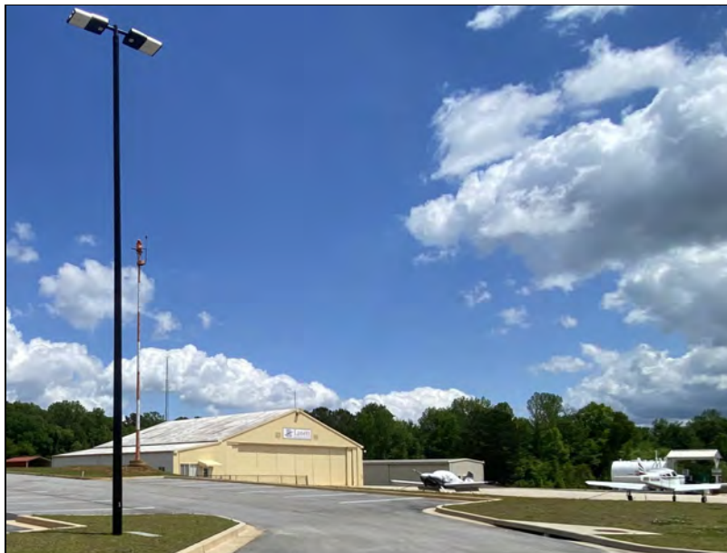
Figure 5.1. Northeast view of hangar facilities.
